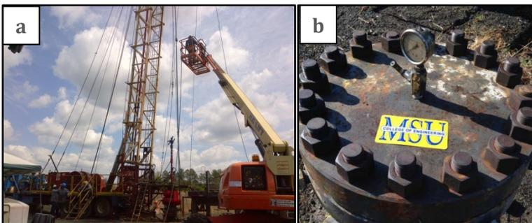
**Figure 1.** a) Filling the bailer with ureolytic microorganisms for delivery downhole. b) 9 5/8" Gorgas #1 well head.
